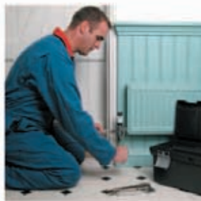
配管工 haikankō plumber
